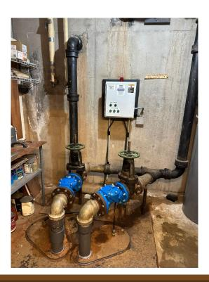
So, next step: two new check valves were obtained and successfully installed and tested last Wednesday (11/15). To effect this, the pit was cleaned out, two new pumps were installed and made responsive to a new control panel, and the job is finished! It has been, it could be said, a long, strange trip, but the system should be good for many years, as was the old one.
