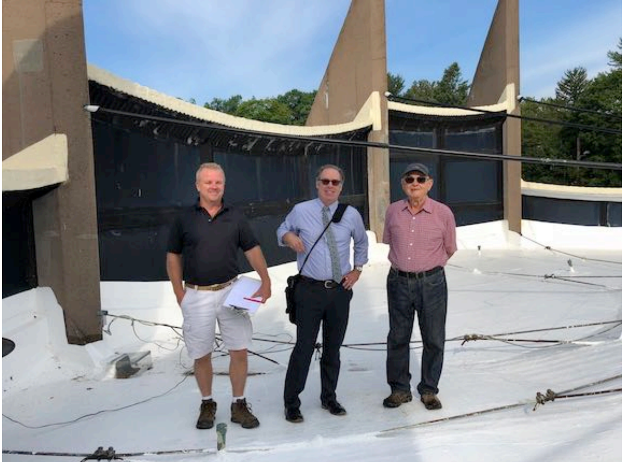
Completed Job - Left to Right, Eagle Rivet Roofing Contractor, Arthur Dias, Architect Hugh Schweitzer and Stu Spence, Chair of B and G
