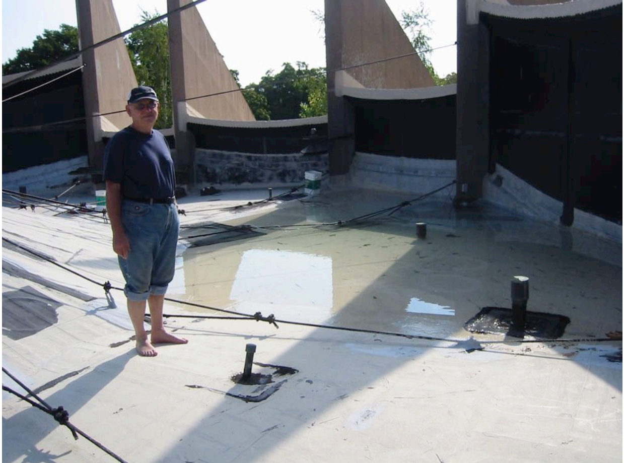
Stu Spence is preparing for wading in a pool to release a controlled flood through the unplugged drain. The pooled water, naturally leaked into the Sanctuary via any defects in the EPDM covering. 2005
