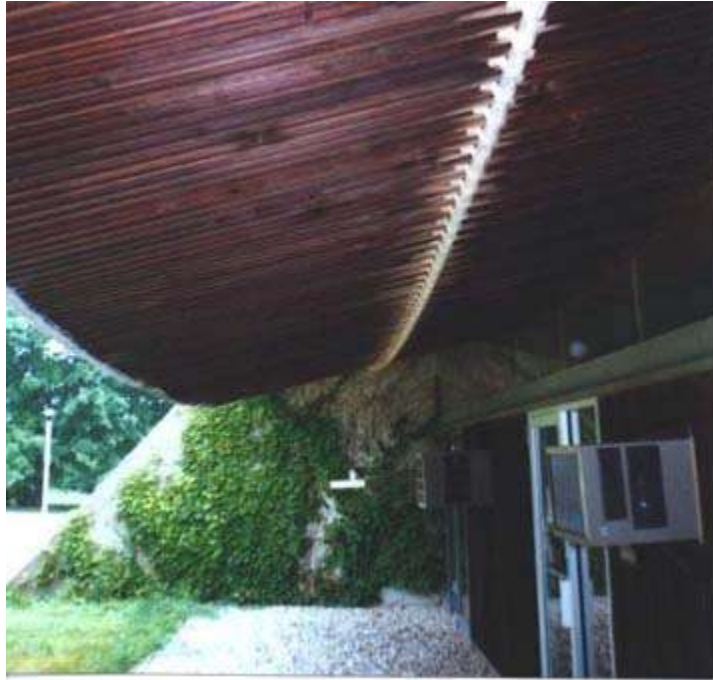
Closeup (from below) of cable-supported roof.
